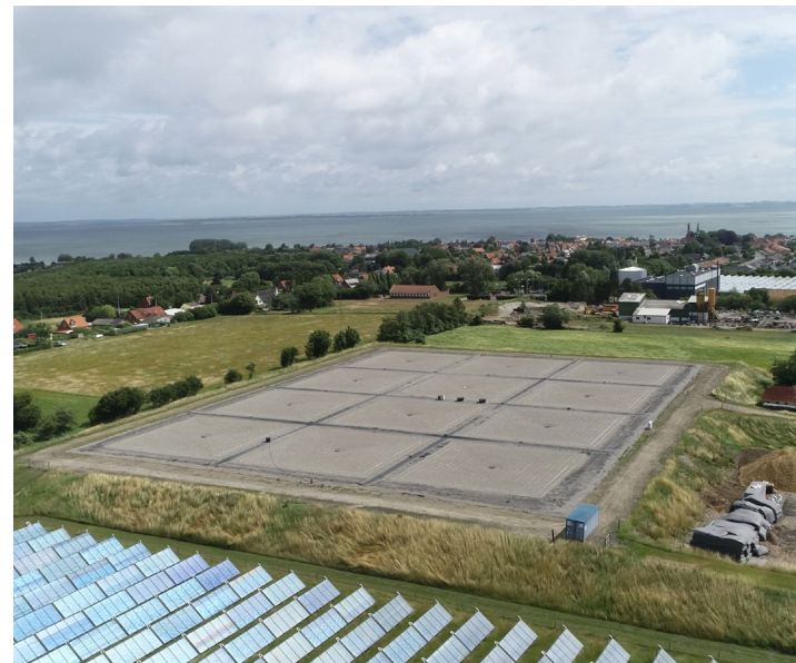
Excess heat from solar heating- or biomass plants and industrial processes as well as excess energy from wind turbines and PV panels can be stored in a PTES for optimum energy utilization and increased system flexibility
